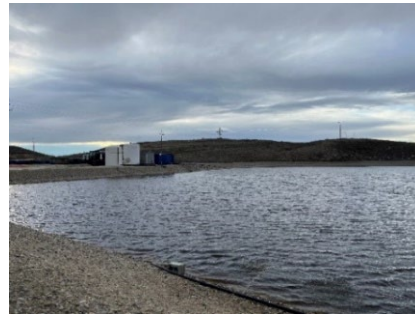
Figure 4: Ada County Landfill Leachate Facility
