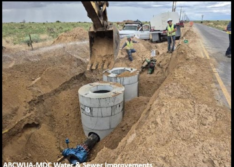
ABCWUA-MDC Water & Sewer Improvements
