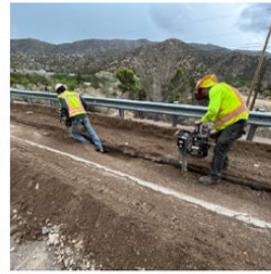
Crew compacted backfill materials.
