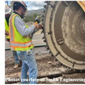
Crew changed out worn teeth approximately every 25' of rock excavation.
