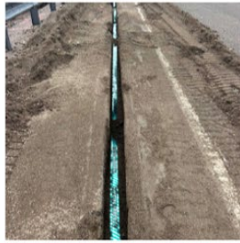
Warning tape placed above the new SAS pipe.
