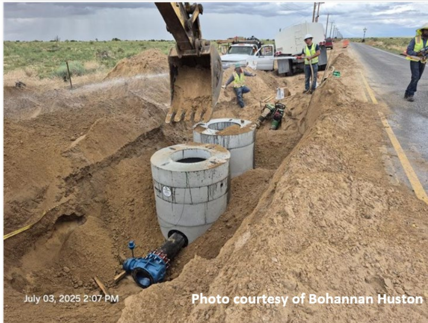
Photo facing North, NMUU completed installing the valve structure and cleanout structure at Sta. 115+00
