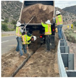
Crew backfilling from dump truck.
