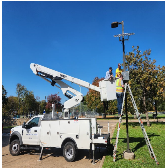
Figure 3. Pod Installation (November 14, 2023)
