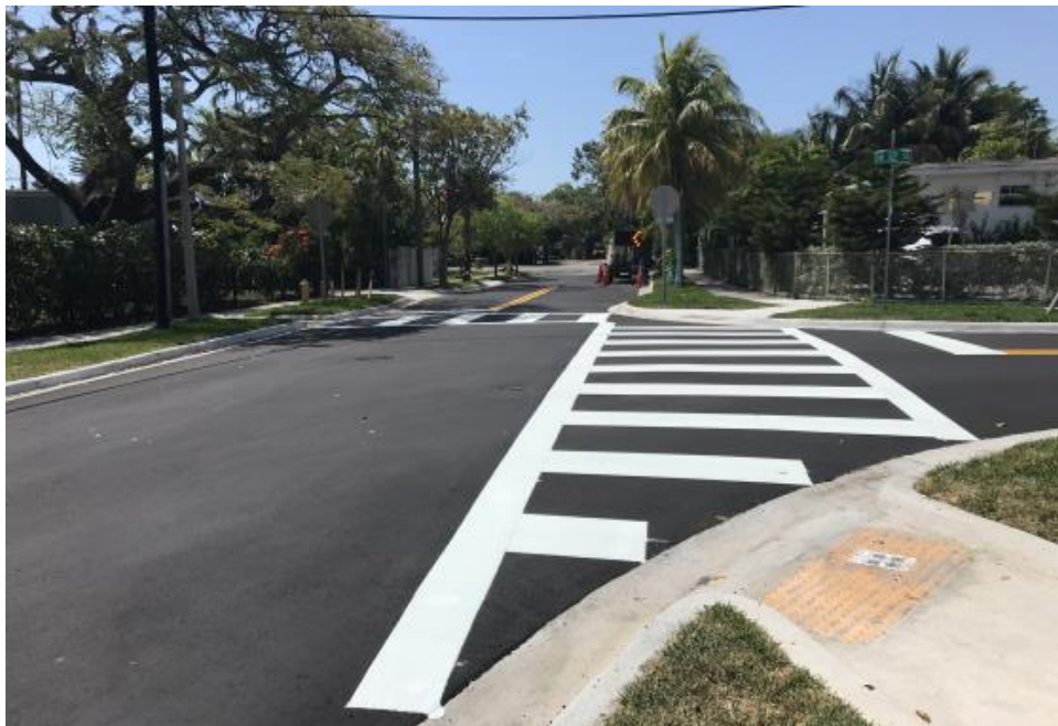
Figure 17 Completed crosswalk with ADA ramps and pavement markings.
