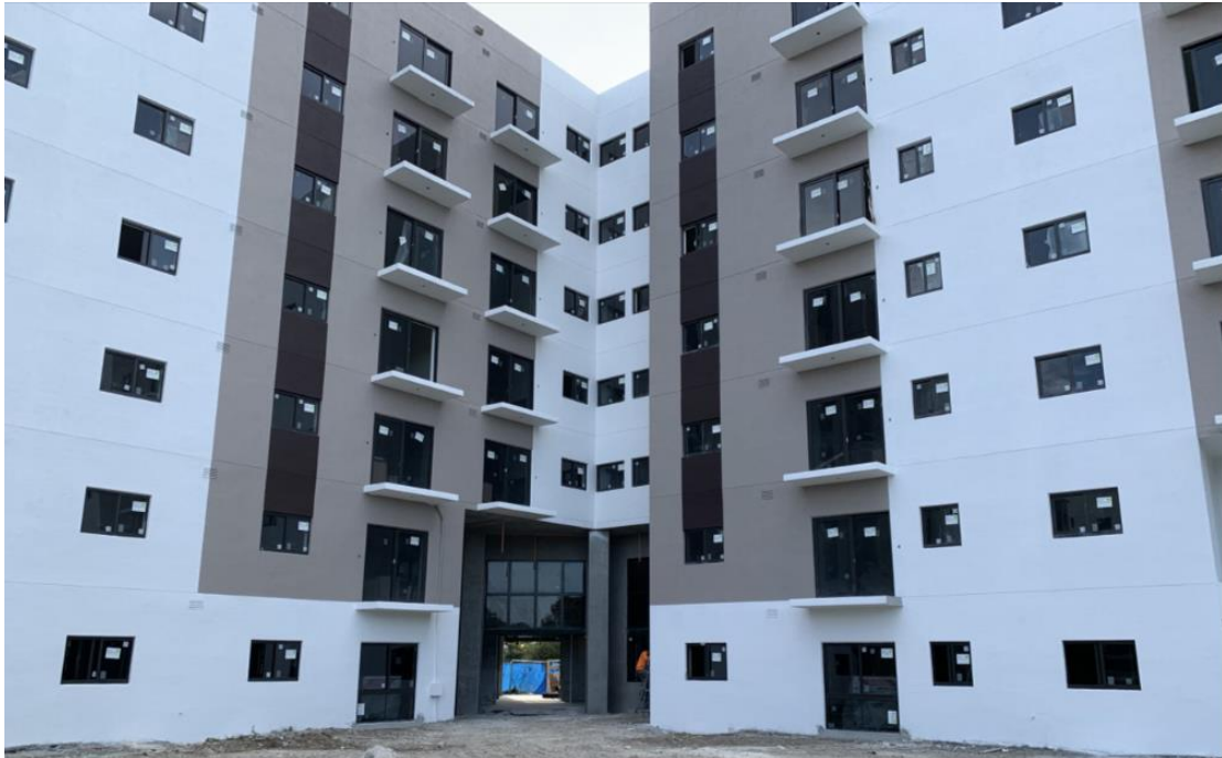
Figure 9 Stadium Towers residential building approximately 92% complete.
