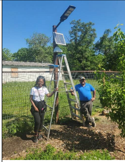
Figure 4. Pod Installation – Joppy Mommas Farm (April 14, 2024)
