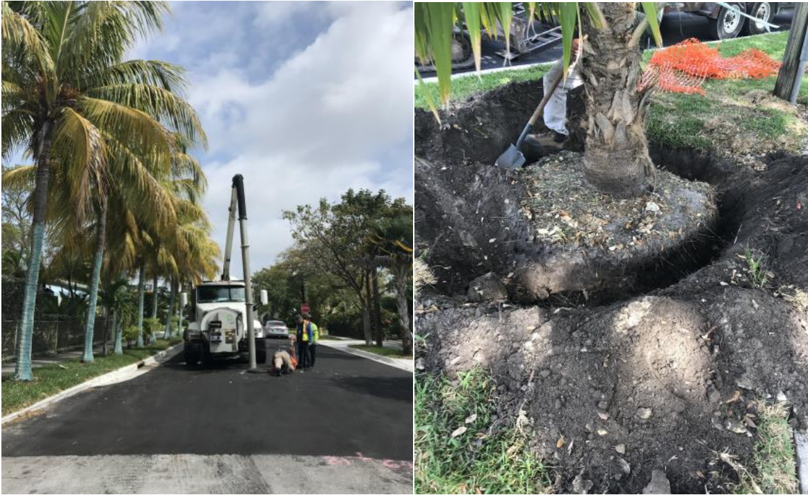
Figure 24: Finished asphalt with drainage work (left); landscaping improvements (right).
