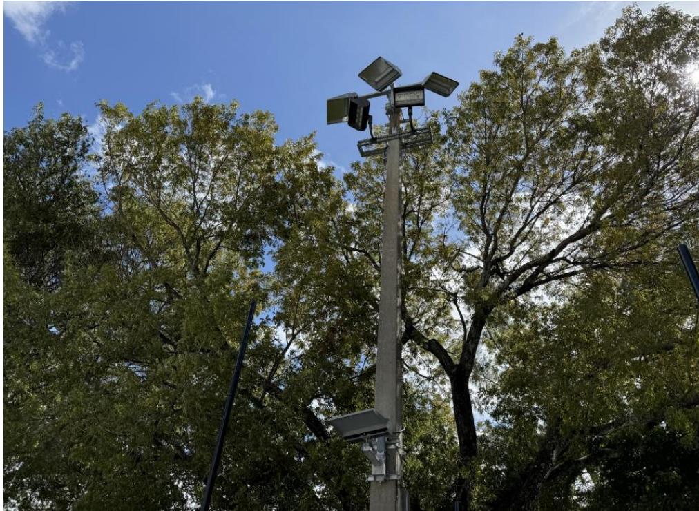
Figure 20: Replaced LED light fixtures on existing concrete posts.
