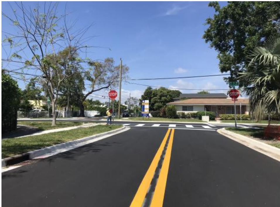
Figure 23: Completed Roadway with pavement markings and curb and gutter.
