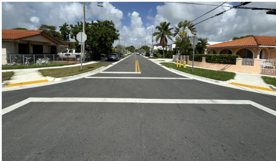
Figure 22: Finished road along SW 24 Terrace.
