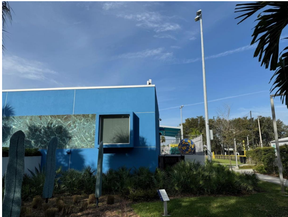
Figure 12: Shenandoah Park Wi-Fi installment (continued) at community center.
