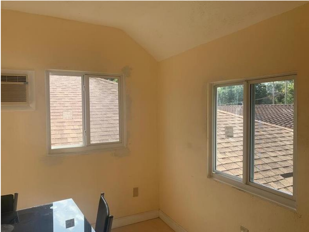
Figure 18: Newly installed impact windows (continued).
