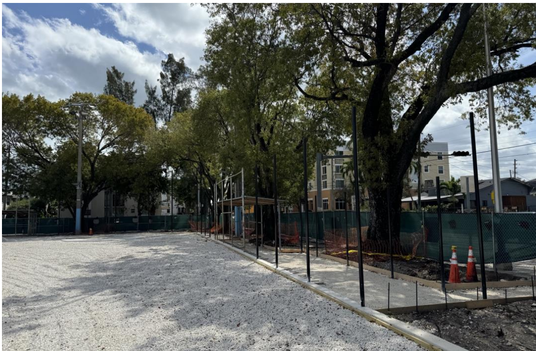
Figure 19: Riverside field turf regrading and curb fencing improvements are in progress.
