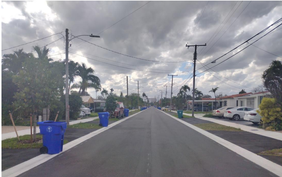
Figure 21: Finished road along SW 25th Street.
