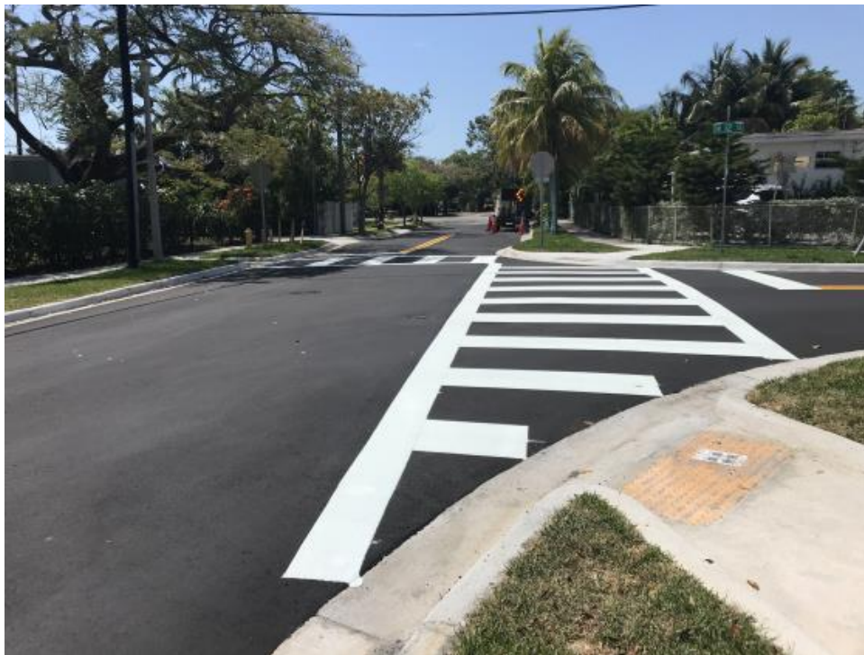
Figure 25: Completed crosswalk with ADA ramps and pavement markings.
