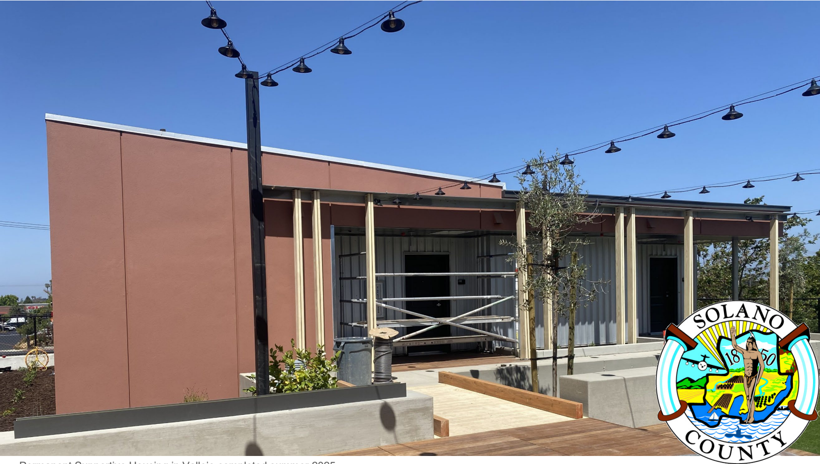
Permanent Supportive Housing in Vallejo completed summer 2025
