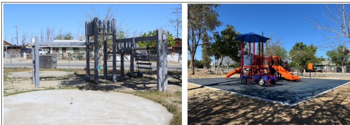
Figure 2-13, Old and New Play Structures at El Porvenir Park
