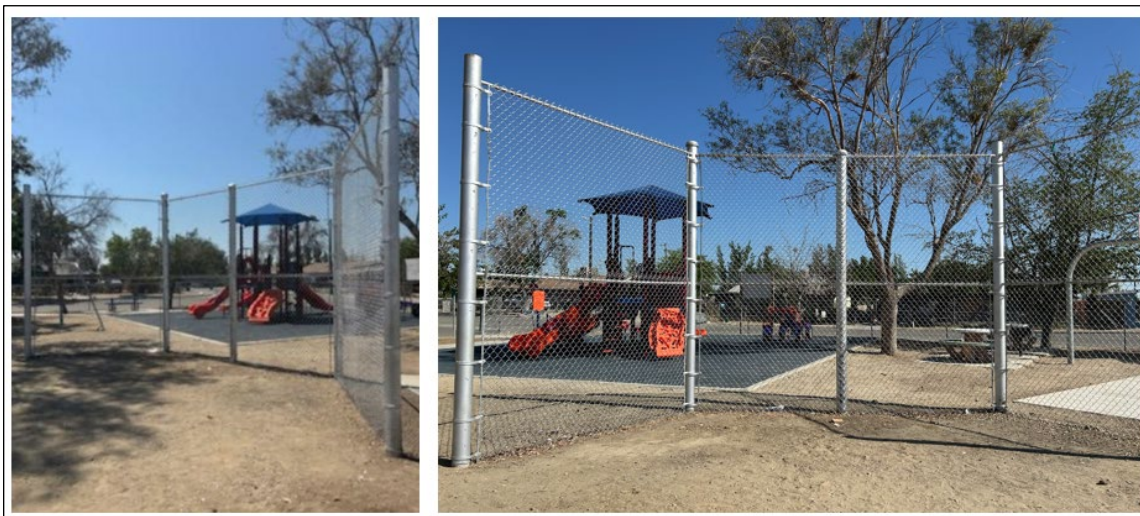
Figure 2-14, Baseball Backstop Repairs at El Porvenir Park
