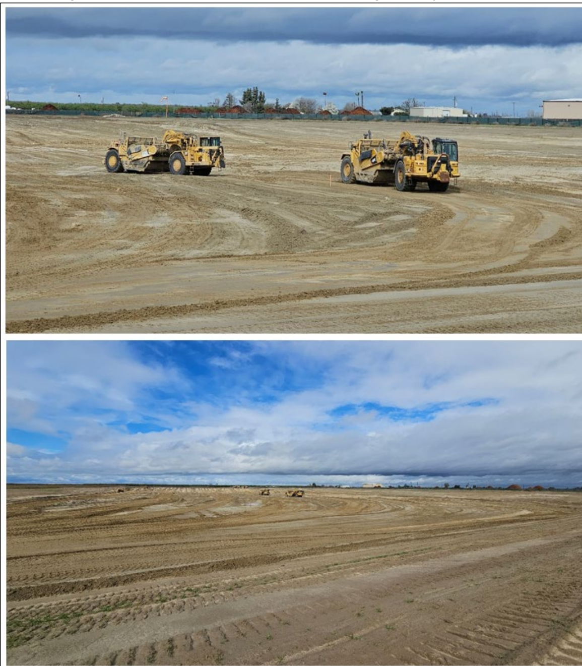
Figure 2-26, Excavation Work at Elkhorn Recharge Facility, March 2025
