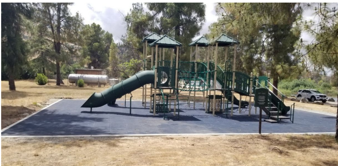
Figure 2-12, New Playground installed at Winton Park
