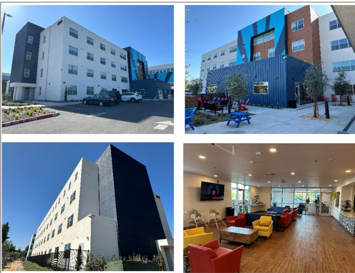
Figures 2-7, City Center Campus, Construction Phase
