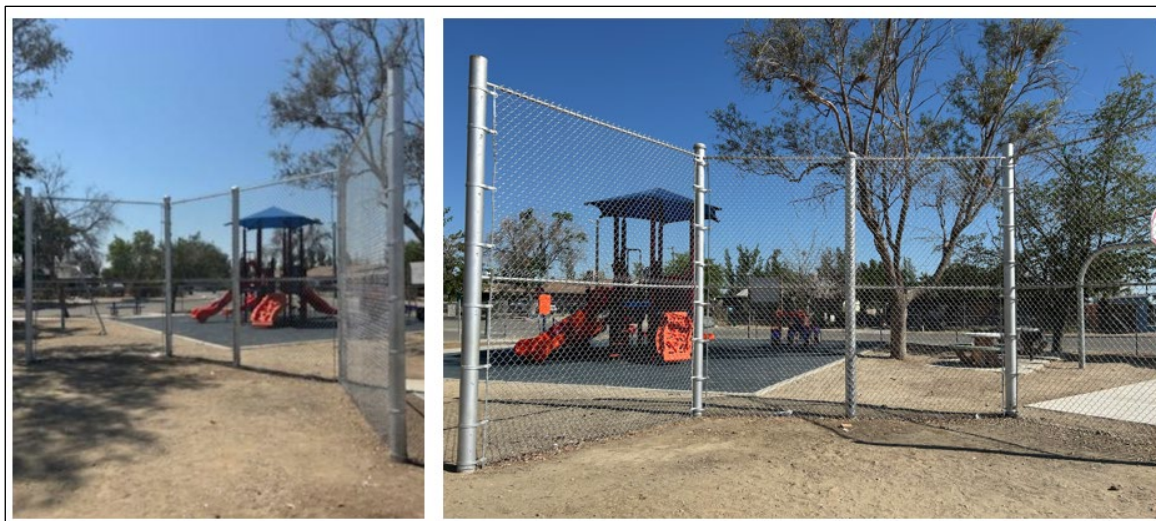
Figure 2-15, Basketball Court Surface Repairs at El Porvenir Park
