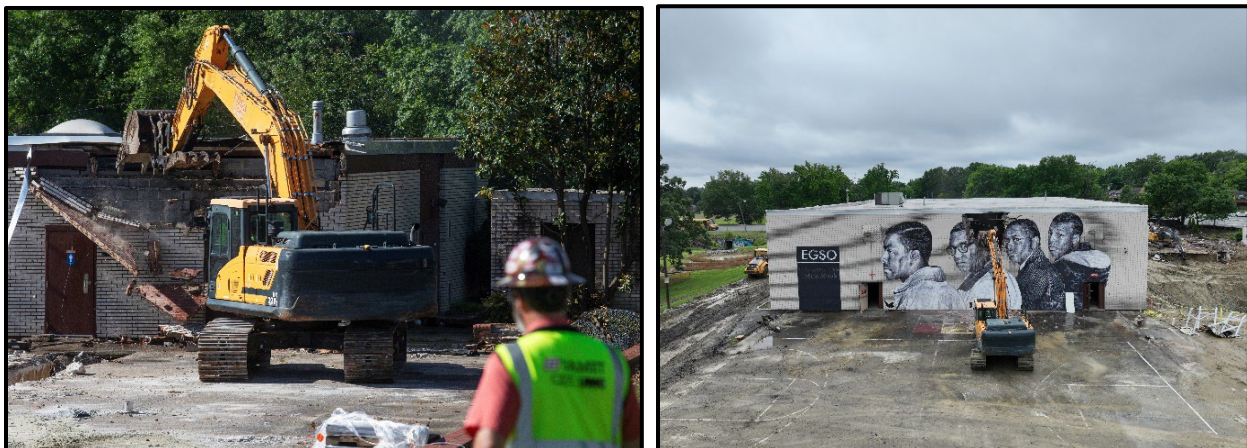
Demolition of Pool, Parking Lot, and Building
