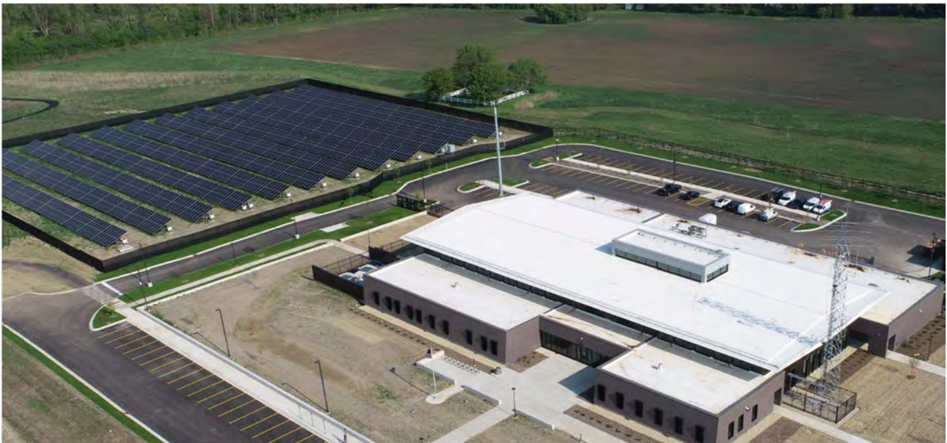
Opening in summer 2025, the state-of-the-art Lake County Regional Operations and communications Facility will serve as a central hub to strengthen 9-1-1 services and emergency response across Lake County. Project [230019]
