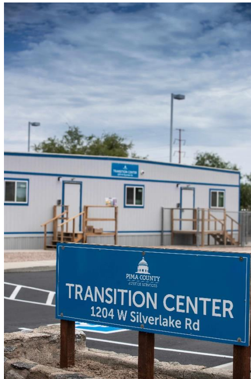
Pima County Transition Center. Photo by Pima County Justice Services.
