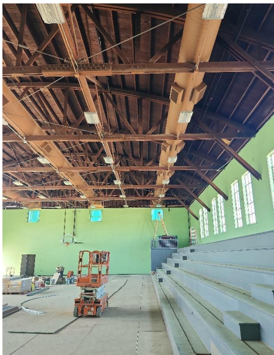
Construction at Curley Gymnasium. Photo by Pima County Project Design & Construction.
