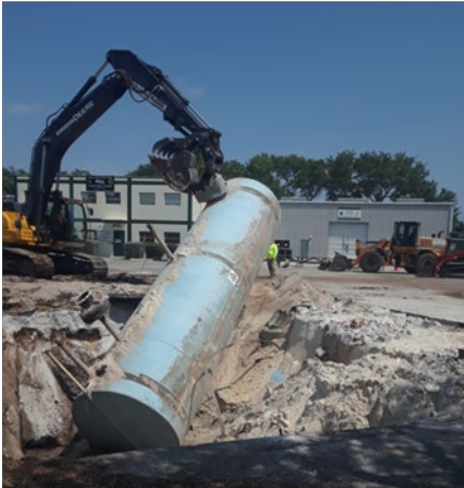
Gas Pump Station Removal
