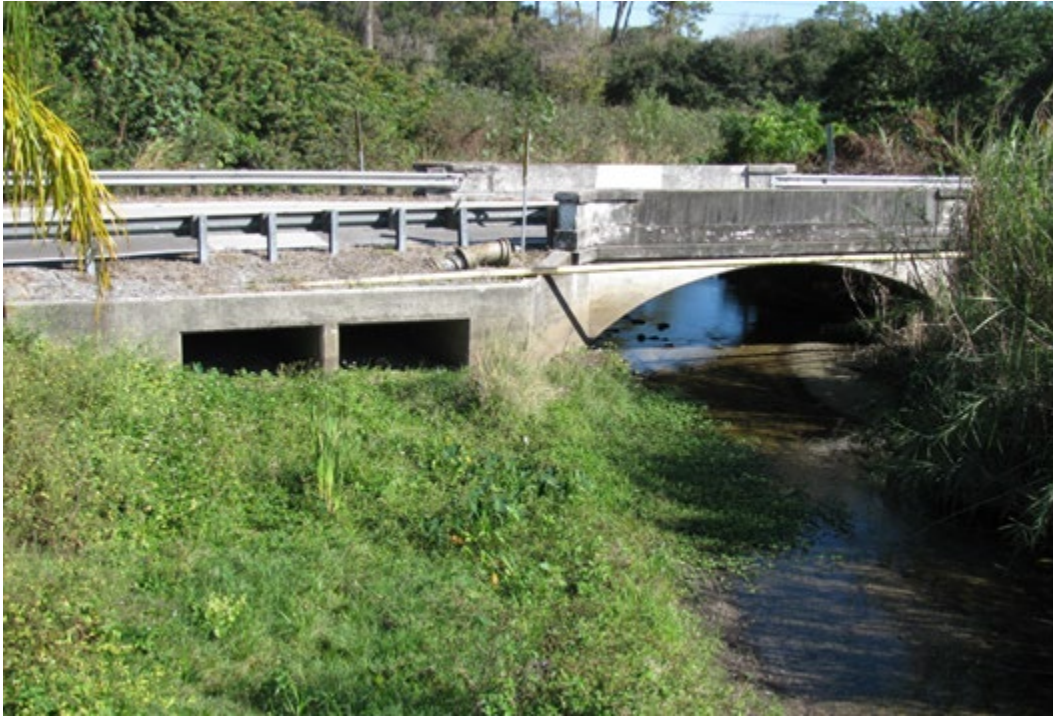
Old Coachman Road Over Alligator Creek Bridge
