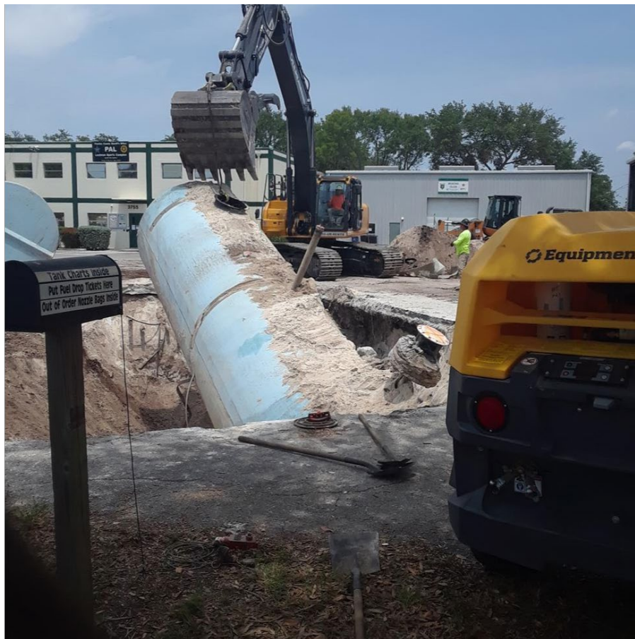
Removal of underground storage tank
