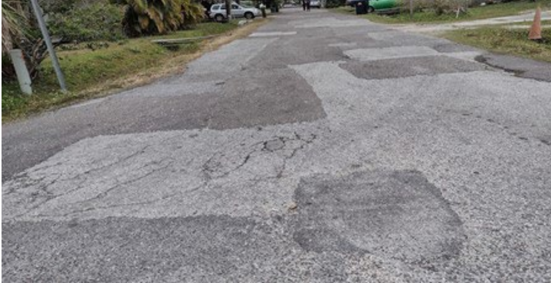
Road included in the Local Group High Point Subdivision improvements.
