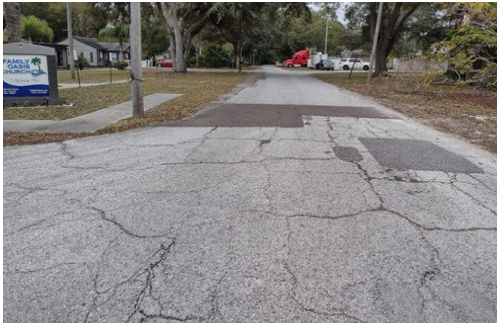
Road included in the Lealman Drainage Improvement project
