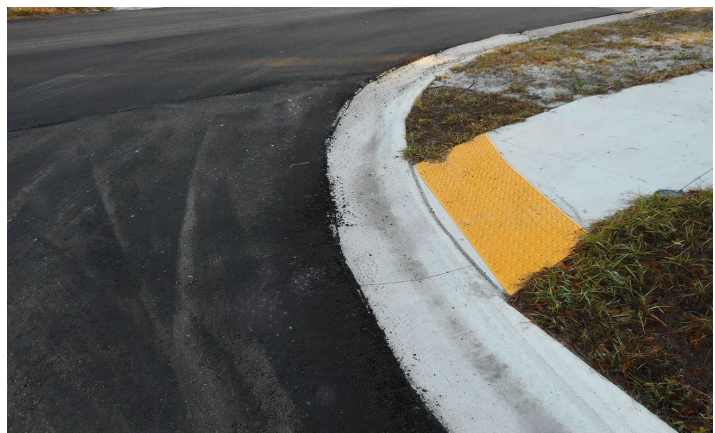
Road included in the Local Group Gulf Terrace & Rainbow Village improvements
