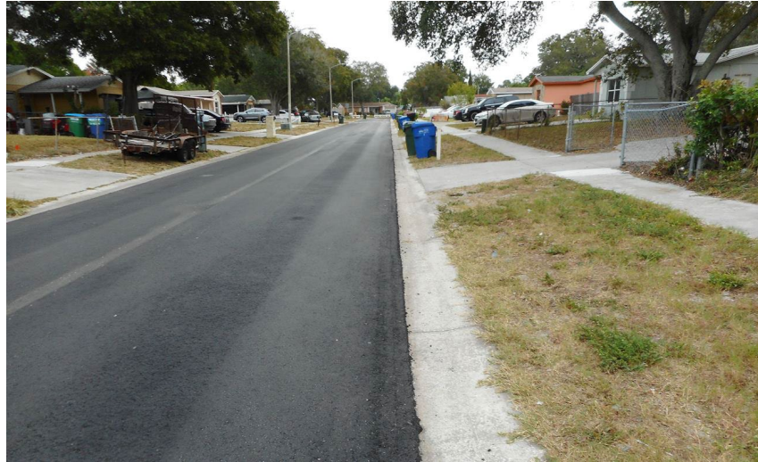
Road included in the Local Group Martin Terrace improvements
