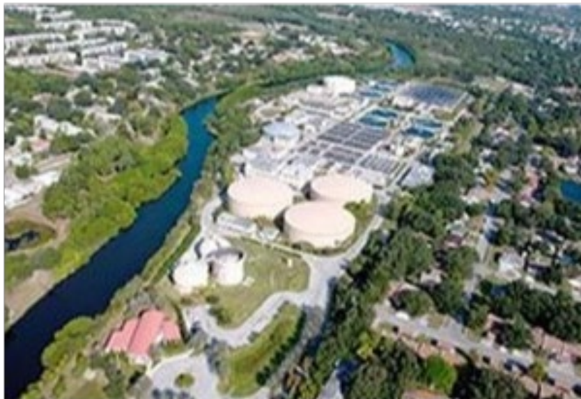
The South Cross Bayou Advanced Water Reclamation Facility (AWRF)
