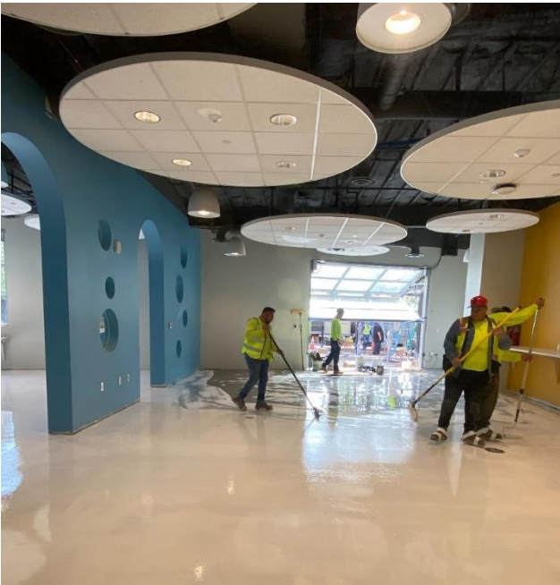
Located on this side of the Library will be the Adult Services collection, public service desk, and staff work area. A garage-style, roll-up door has been installed to promote patron flow to the outdoor activity patio.
