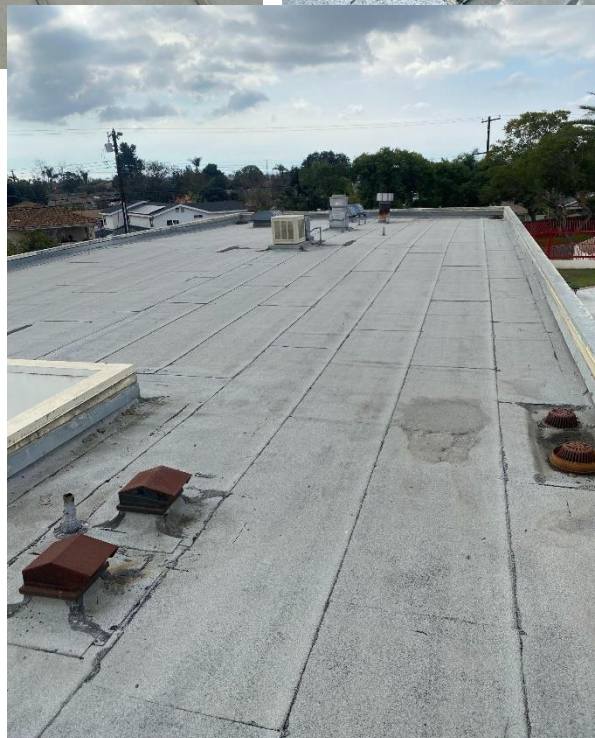
Images from the Salgado Center Renovations.
