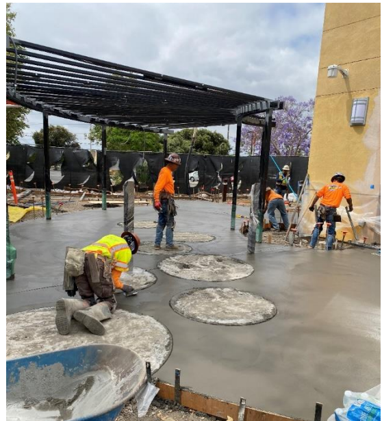
Construction of the outdoor activity patio is nearly complete. The space will include shaded public seating, amphitheater-style seating for Library programs, as well as a children's play area.
