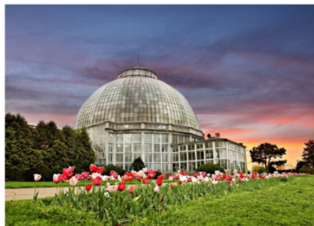
FRF is being used for a major renovation of the Anna Scripps Whitcomb Conservatory on Belle Isle, Detroit
