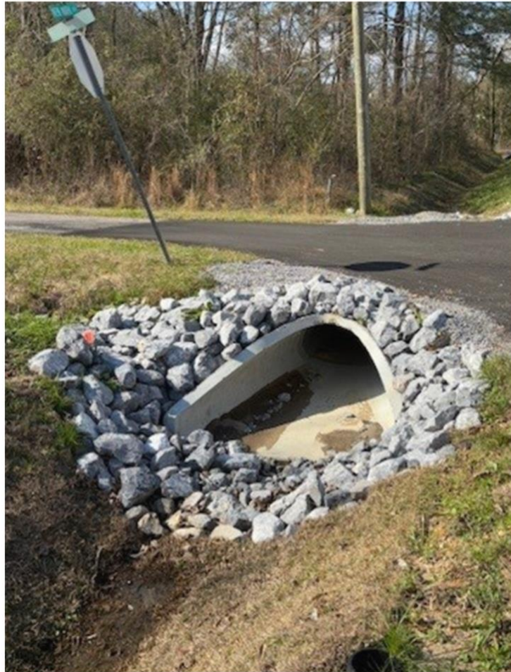
City of Sumrall: Stormwater Upgrades
