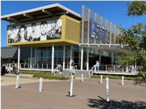
Safety Bollards Before
