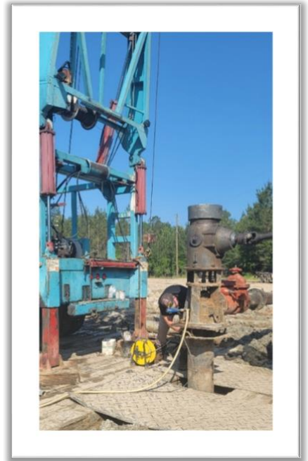
Potable Water Supply Well in Construction
