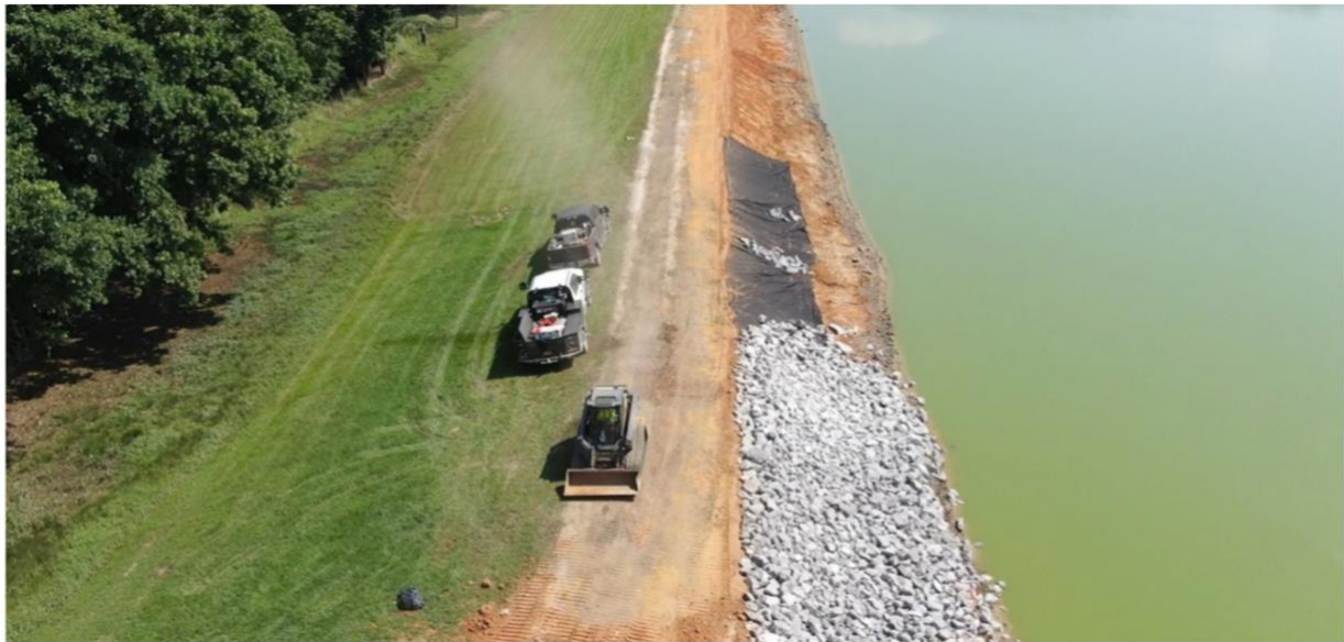
City of Philadelphia: Wastewater Treatment Lagoon Project
