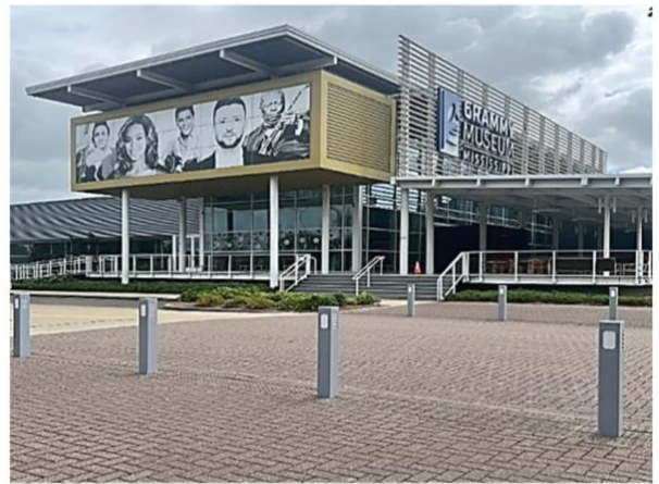
Safety Bollards After
