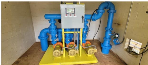
Booster Station Nearly Complete
