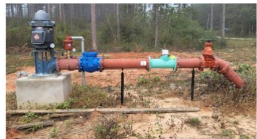
Potable Water Supply Well in Construction
