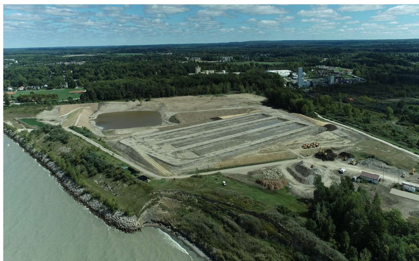
Fairport Harbor after Construction
