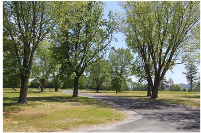
Paving completed at Shawnee State Park
