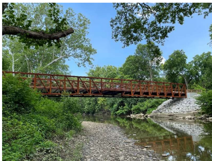
O'Bannon Bridge in Little Miami State Park
