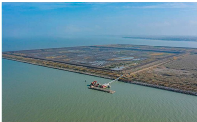
Aerial view of Toledo Harbor Dredge Facility
