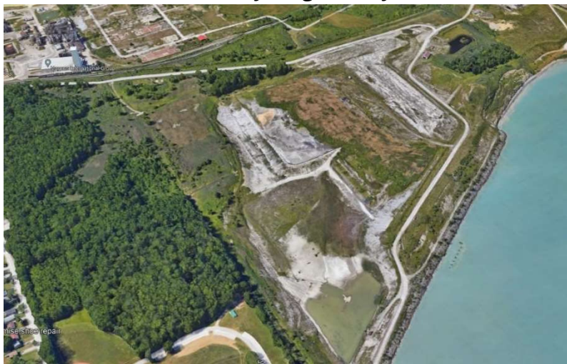
View of Fairport Harbor Site Before Construction
