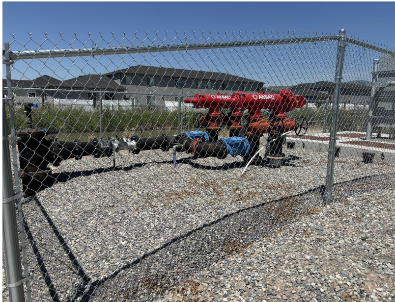
Figure 3. Tremonton City's Secondary Water Project.
