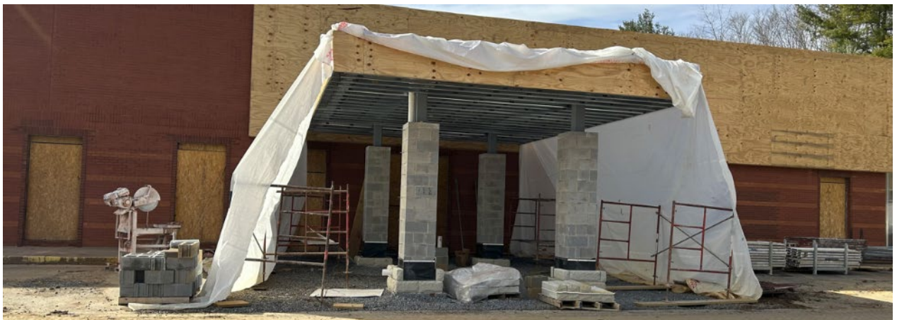
Actual Main Entrance Under Construction
