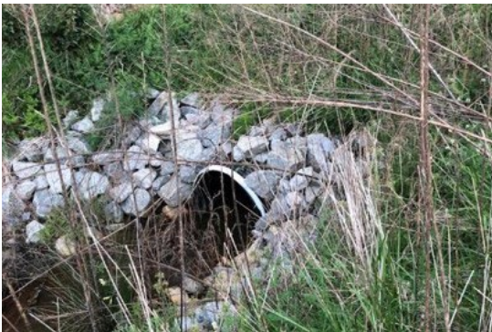
City of Emporia (440-203): Completed drainage culvert.
