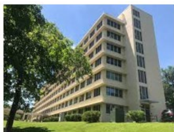
720-18576-24-02 Catawba Hospital HVAC replacement
