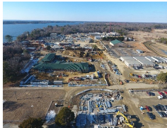
Hampton Roads Sanitation District (440- 304): Overview of construction site at the James River Wastewater Treatment Plant.
