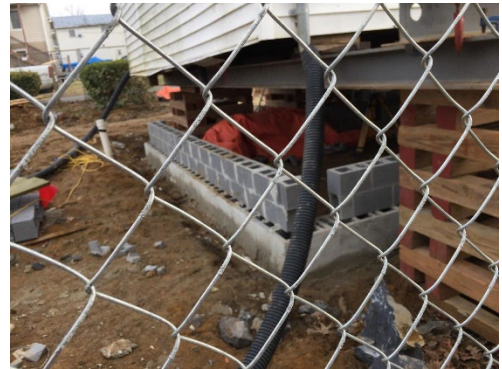
The renovated foundation
