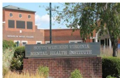
720-18576-05-01 SWVMHI HVAC replacement
