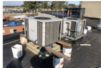
720-18576-29-02 PGH HVAC replacement
