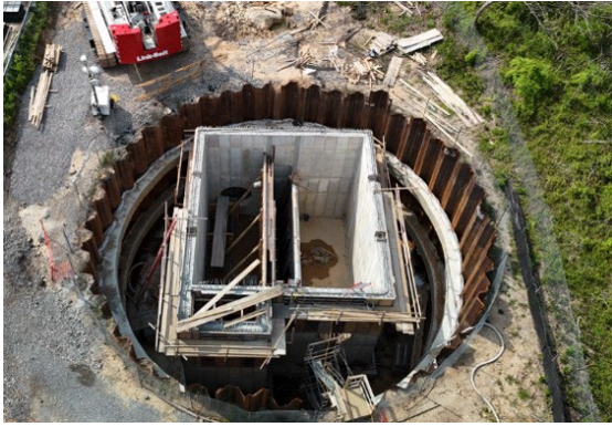
City of Richmond (440-102): Phase 3 of Chimborazo Combined Sewer Outflow improvements
