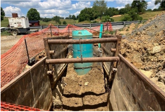
Washington County Service Authority (440-237): Halls Bottom Road manhole install
