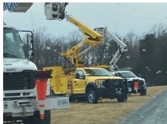
Bucket trucks in Thomas Jefferson Planning District Commission project with ISP, Firefly Fiber Broadband
