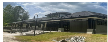
New High Bridge Trail State Park Visitor Center
