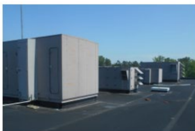
720-18576-94-01 VCBP RTUs (rooftop units) replacement
