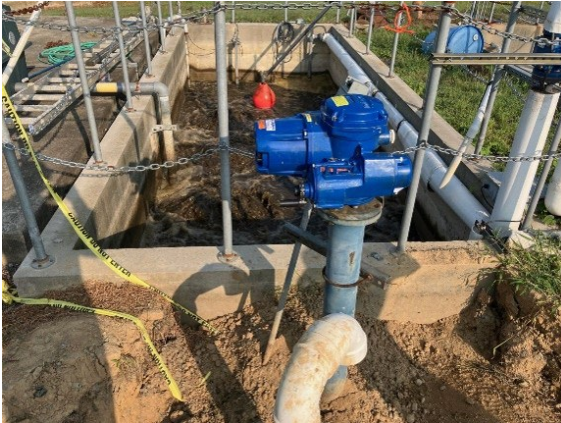
Town of Parksley (440-408): Completed SBR plug/valve repair
