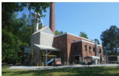
720-18576-29-11 PGH Boiler Plant upgrade
