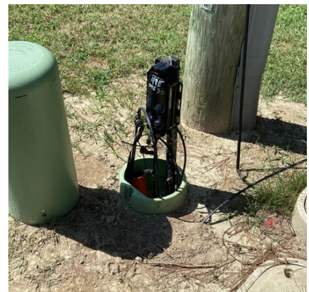
A broadband network terminal, where lines are connected between line extensions to households and mainline broadband infrastructure
