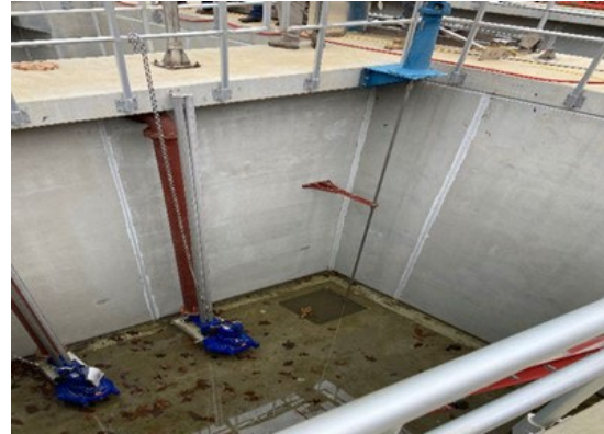
Nelson County Service Authority (440- 214): Installed pre-aeration membrane bioreactor tanks.
