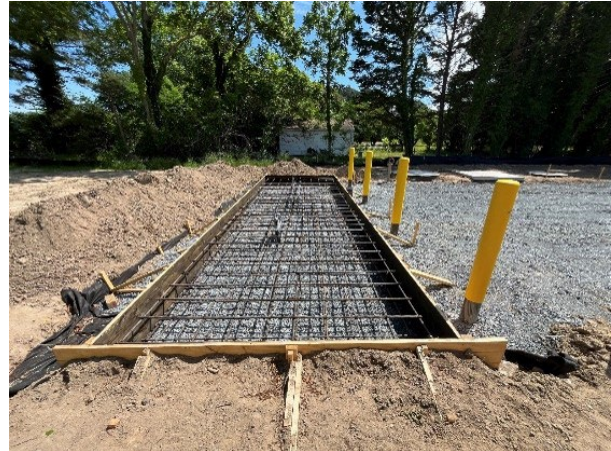
Town of Accomac (440-404): Pump station work
