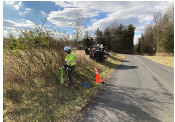
Last mile fiber optic construction in Middlesex County project with ISP, All Points Broadband
