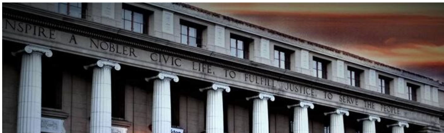
Figure 2: Stockton City Hall
