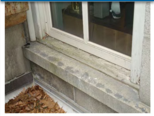
Fig 2: Typical Rotten Windowsill
