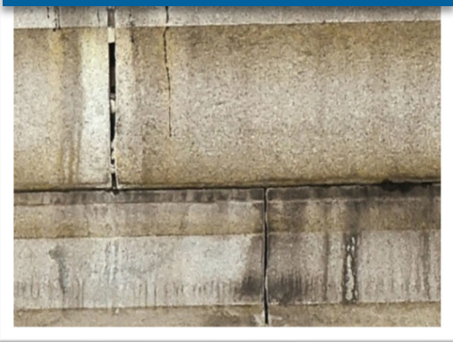
Fig 1: Open Joints, Failing Masonry
