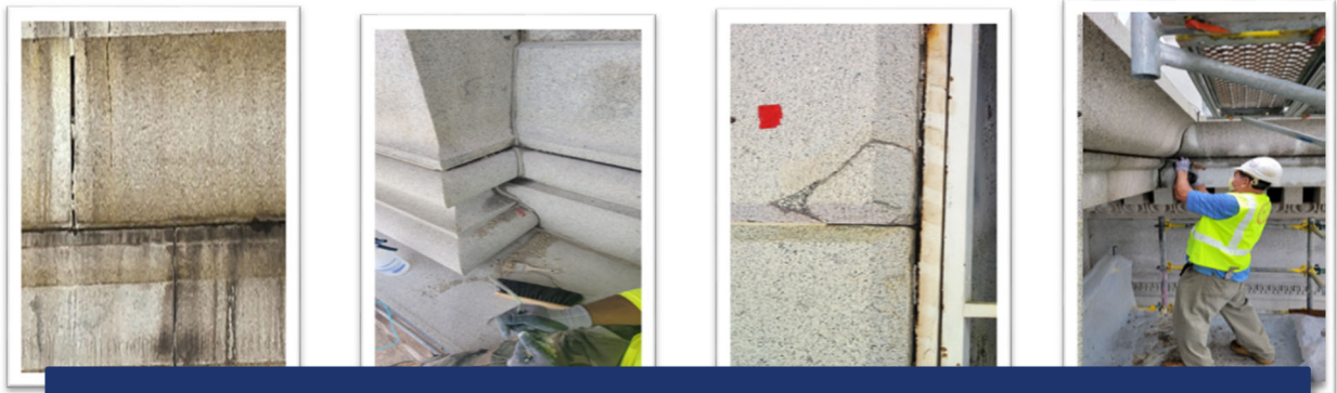
Figure 1: Open Joints, Failing Masonry
