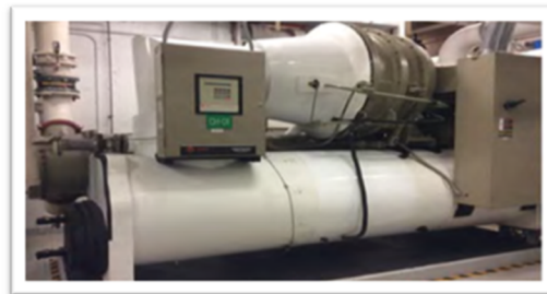
Centrifugal Chiller Plant (1 of 4 chillers pictured above)
