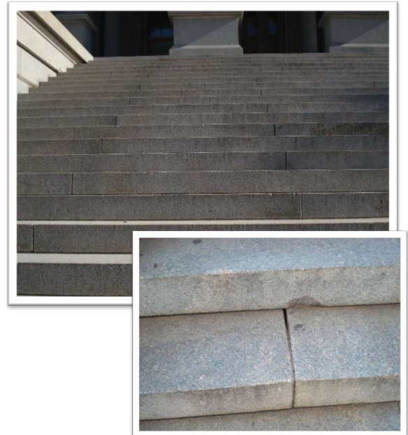
Close up view of missing/loose sealant at portico steps
