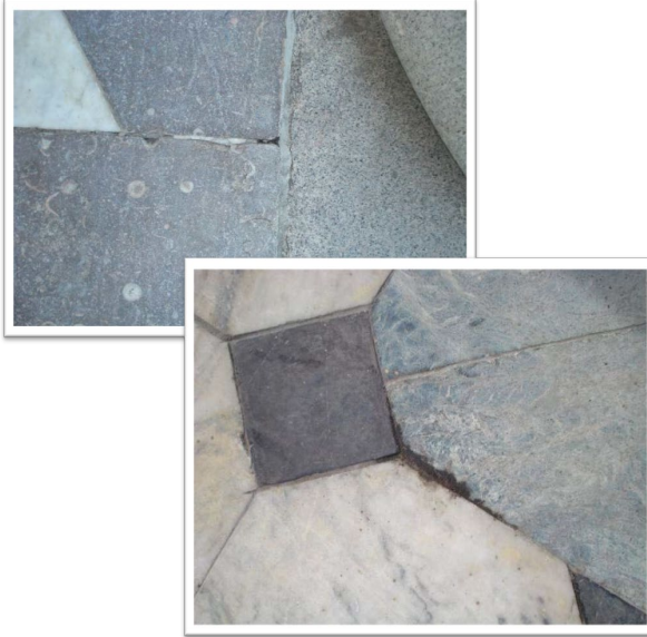
Typical portico grout joint deterioration and moisture leach
