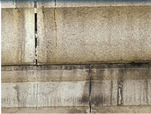
Fig 1: Open Joints, Failing Masonry
