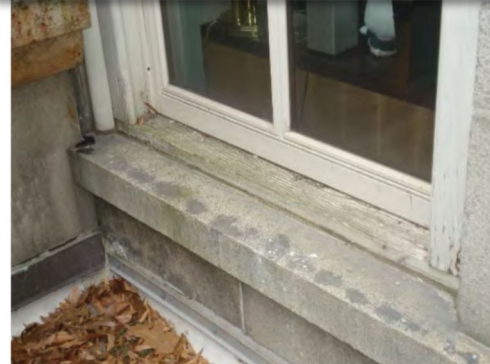
Fig 2: Typical Rotten Windowsill
