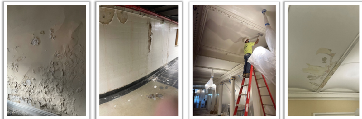
Figure 5: Wall and Finish Deterioration; Interior Ceiling
