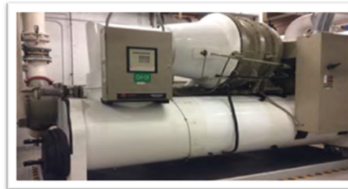
Centrifugal Chiller Plant (1 of 4 chillers pictured above)
