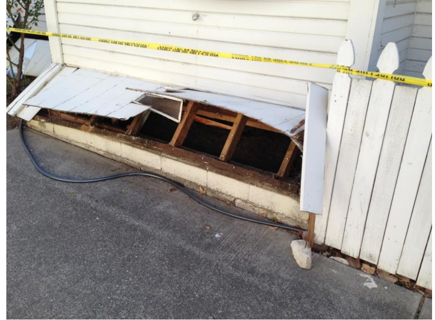
Cripple wall collapsed
